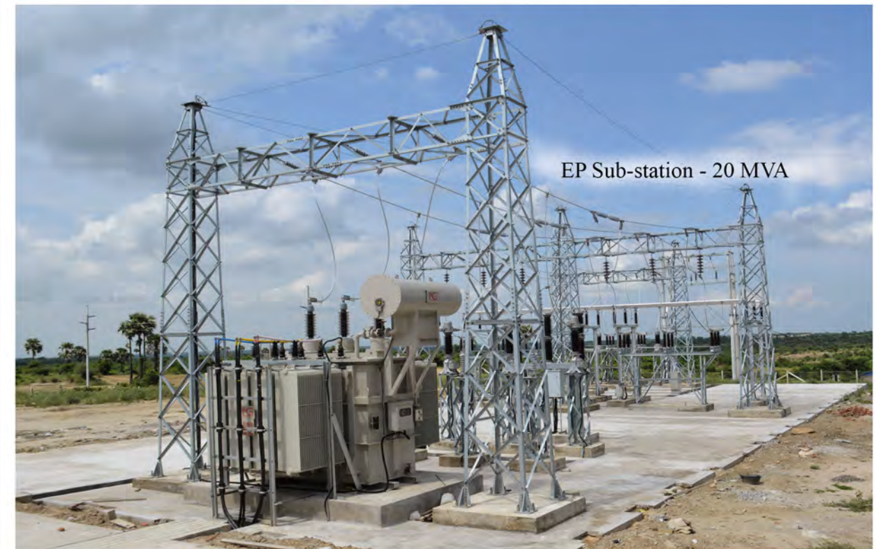
Solar Power Plant & 20 MVA Sub-station
