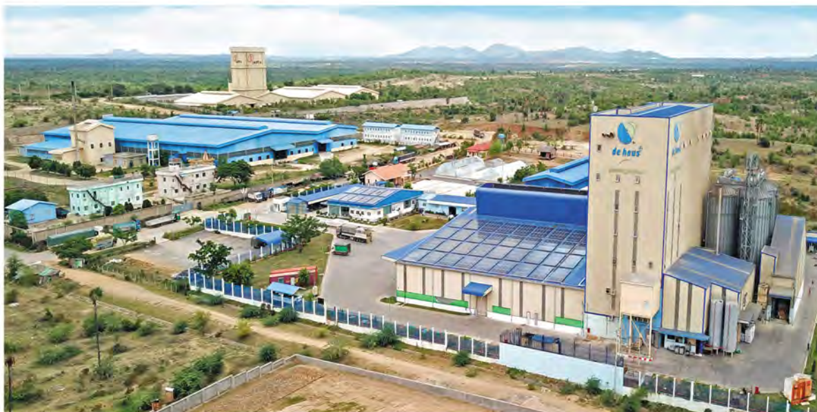
Deheus Feed Mill Factory - Netherlands
